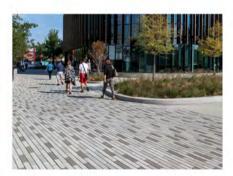
Permeable Pavers + Porous Asphalt
